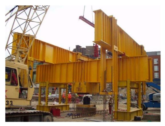
Figure 5.1 30MN reaction pile test
