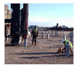
Figure 5.8 Dynamic load testing of driven precast concrete piles
